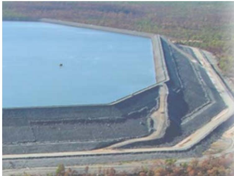
An example of side hill containments is the Cluff Lake Waste Management System, where an embankment was built with a compacted soil/bentonite layer beneath and parallel to the inner wall surface that was keyed into the foundation material.
