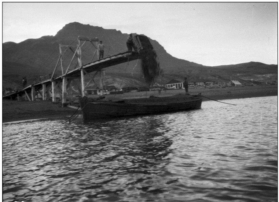
Photo 2. The loading ramp, anno 1930. The coal was loaded into barges and sailed to ships anchored further from the coast. Photo: Copyright Danish Arctic Institute.
